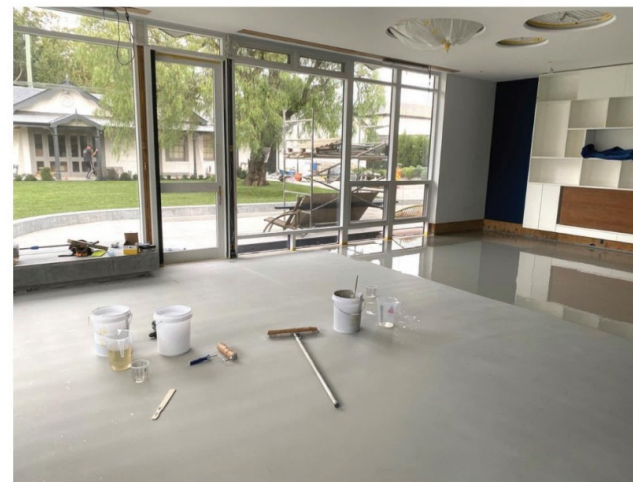
Above: Surface Preparation
