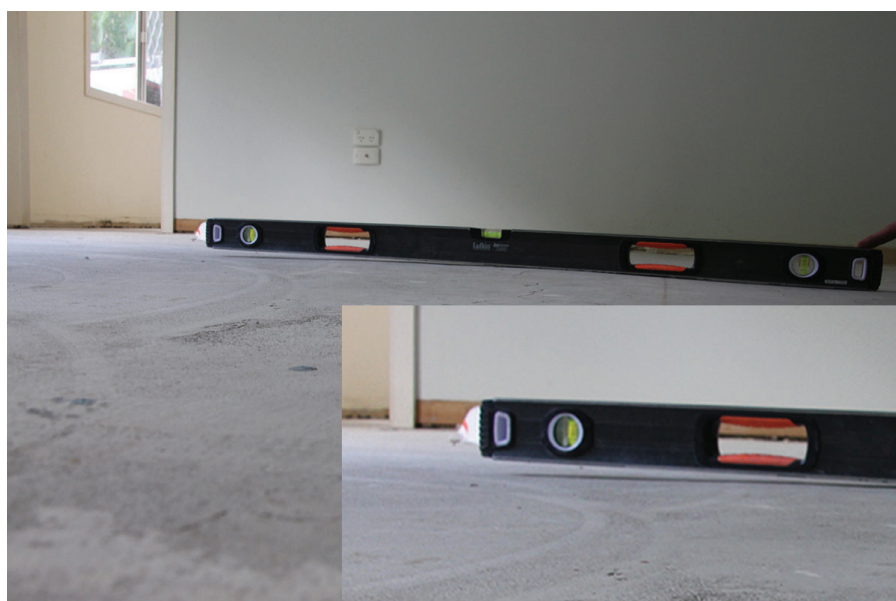
Above: Concrete Slab Flatness
