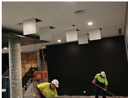
Above: Busy Worksite
