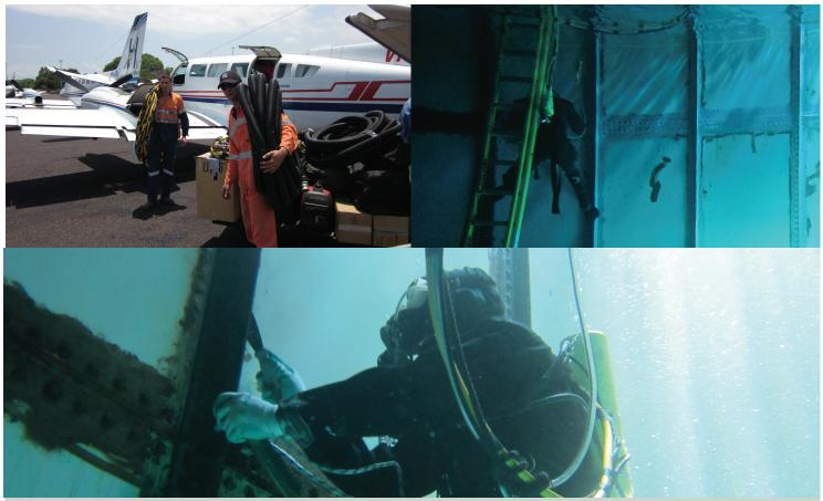
A remote island community in the Arafura Sea were running out of drinking water on a regular basis due to severe leaking in their main storage tank. The original sealing compound had failed and the tank was now leaking from just about every seam.
