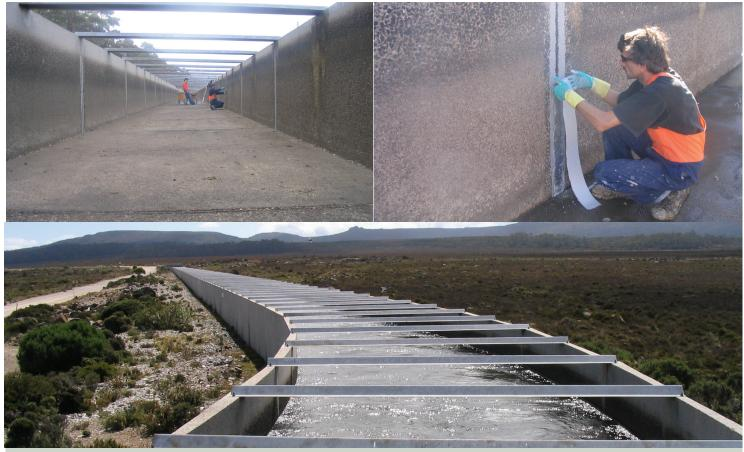
Hydro Tasmania was searching for a product to seal the 2,700 lineal metres of expansion joints in the Fisher Flume (a main water channel in their hydroelectricity scheme). The main concern with such a vital artery was minimising shutdown, which meant they were after a sealant that could handle the unpredictable conditions during installation and remain flexible when the temperature approached freezing in the winter months.
